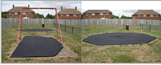
Swings and Round-about removed and safety surfacing partially missing
